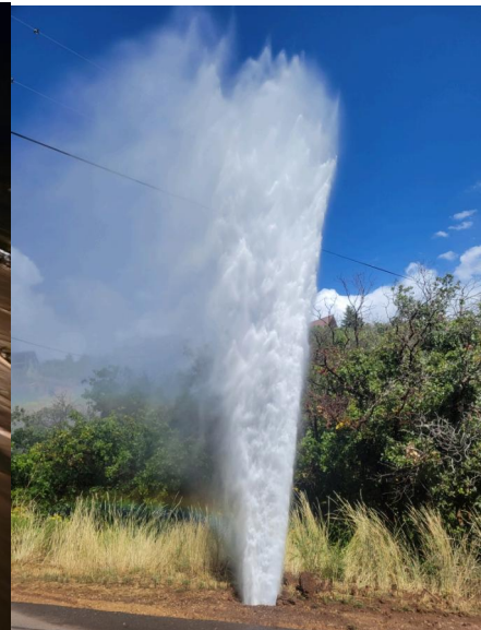
St. Moritz Water line break – 9/15/24
