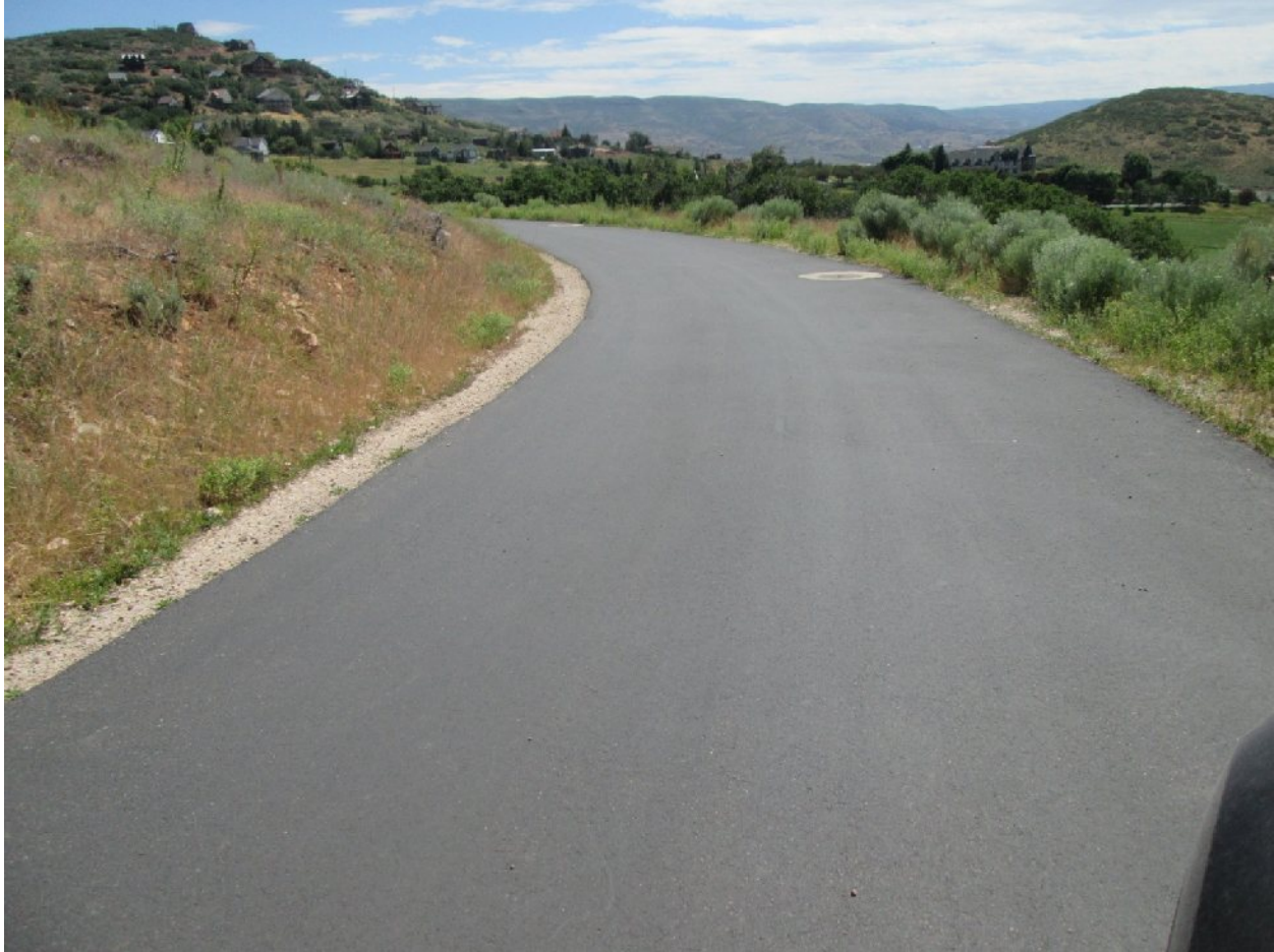
Photo 3. Very Good Condition – Luzern Rd from Luzern Rd to Luzern Rd (RSL = 14 years)
