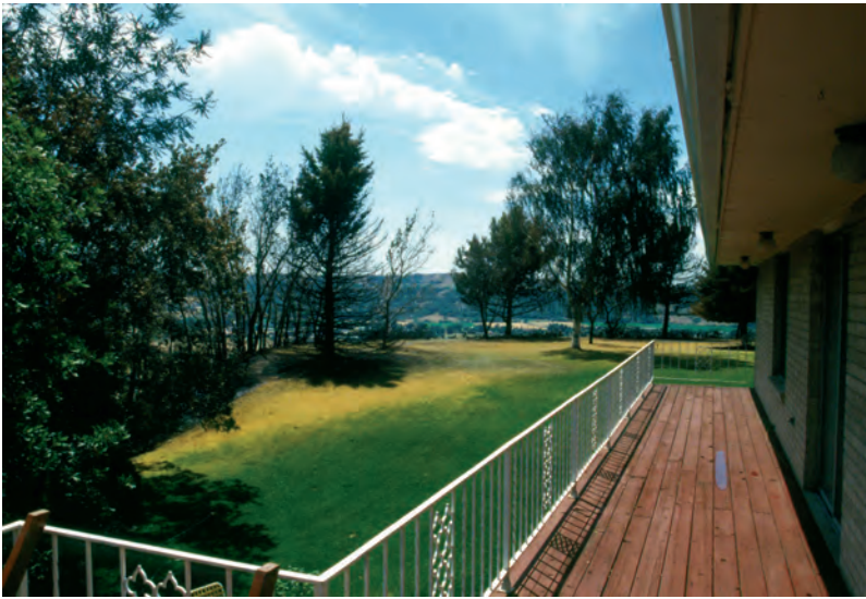
This home's green, moist vegetation and setback from the hillside prevented it from igniting in the fire that burned up the hill. The wooden deck is a problem, and should be replaced with non-flammable material.
