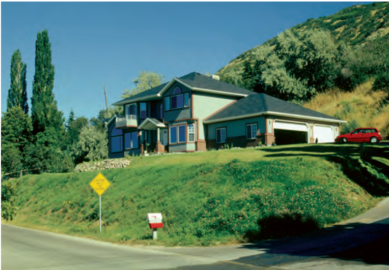
This home has good, wide firewise landscaping within much of its home ignition zone. Its Zone 2 is “clean and green”.
