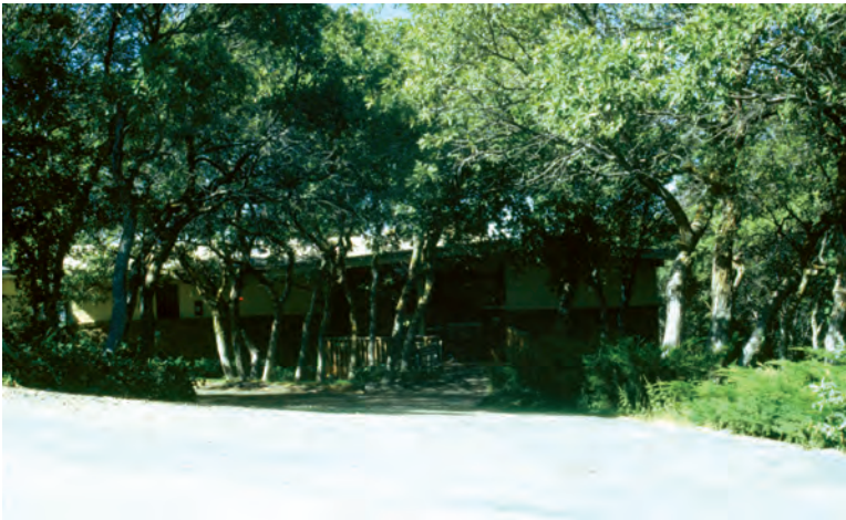
Although this home close to the road, its Zone 2 landscaping is not firewise, with highly flammable oak trees overhanging the roof.
