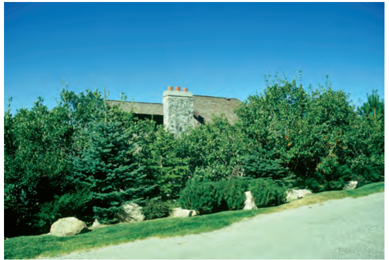
Continuous fuels and a wood roof increase this home's risk for damage from a wildfire.
