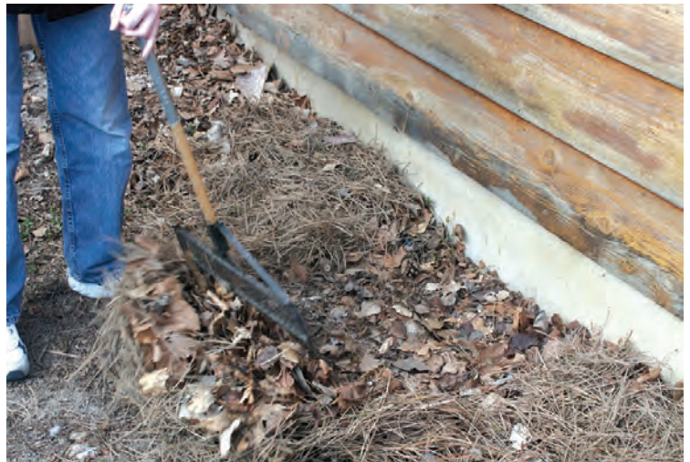
Rake and remove dead leaves, needles and other flammable debris from near structures.
