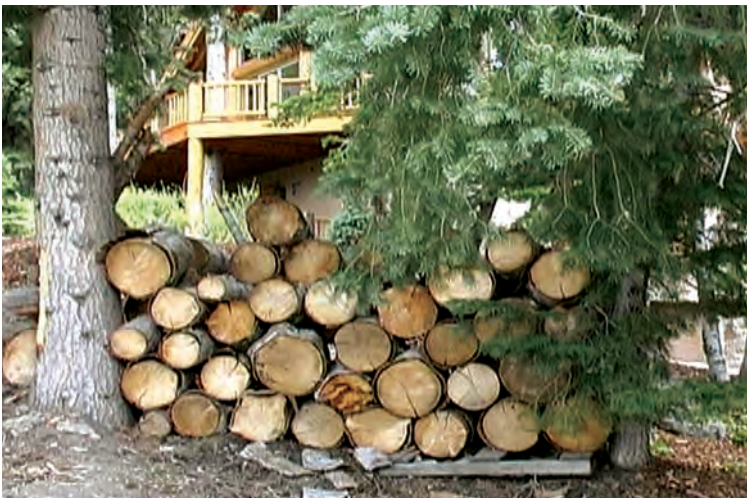
This wood pile should be moved at least 30 to 100 feet away from the house. Notice the unenclosed deck and tree growing up through the deck – both increase risk from a wildfire.
